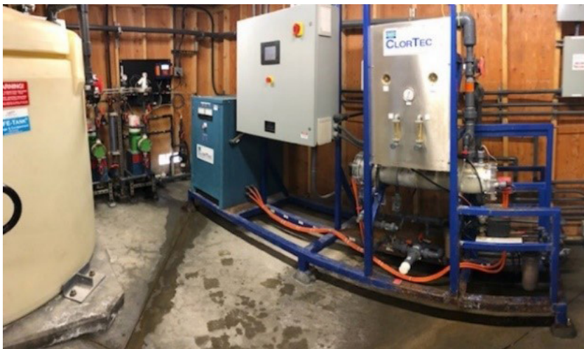
Old Chlorine Generator
