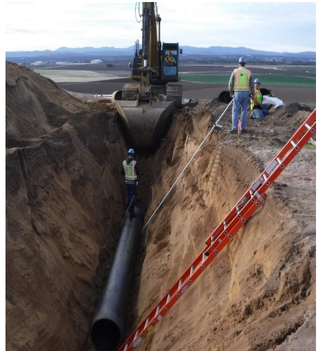
Construction of the MCWD's RUWAP Transmission Pipeline that will serve both MCWD customers and M1W's Pure Water Monterey Project which was recently completed.
